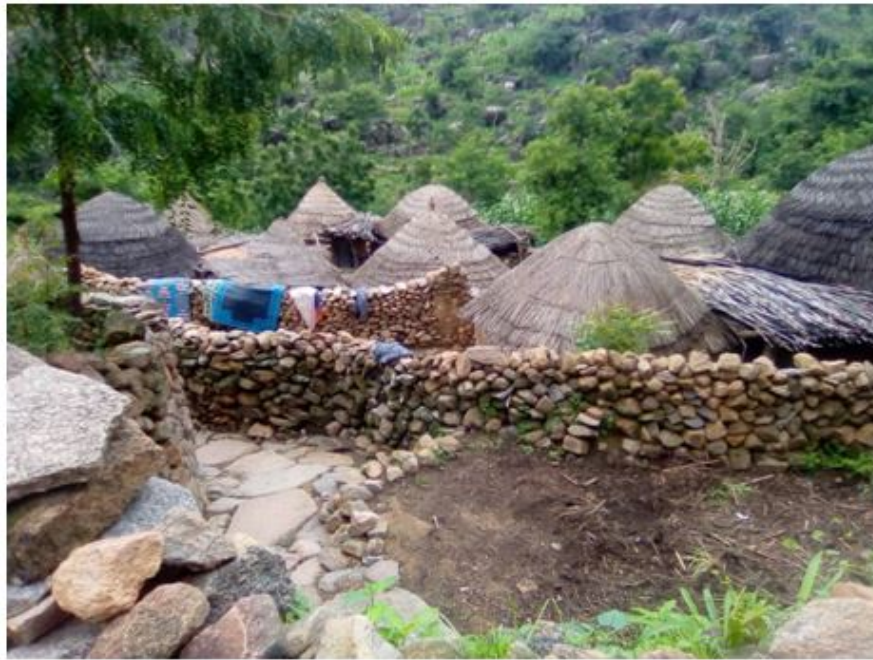
Picture 3: Stone Dwarf Wall with green vegetation Source: Sham Anthony (Site Manager), 2021
