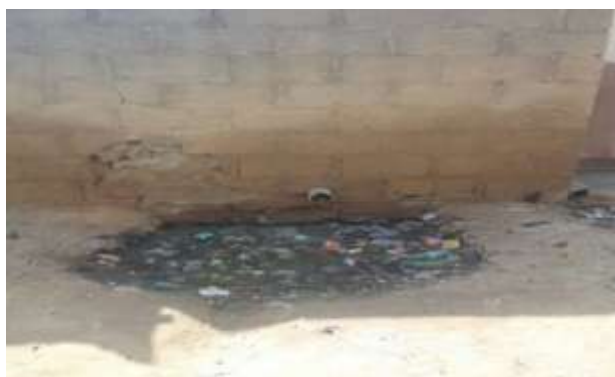
Plate 4: Dug pit for disposing grey water in Gamboru ward
