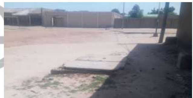
Plate 1: Soak-away Sited on Road Reserve in Bolori I Ward
