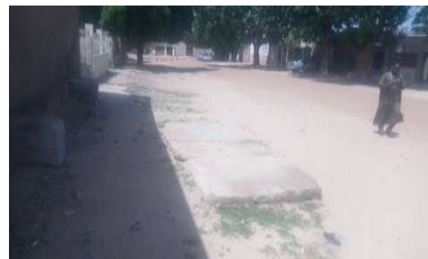
Plate 2: Soak-away sited on road reserve in Gwange III Ward
