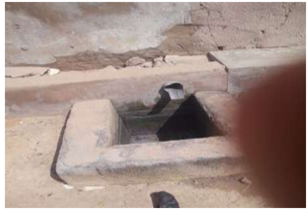
Plate 5: Paved pit for disposing grey water in Bolori II ward
