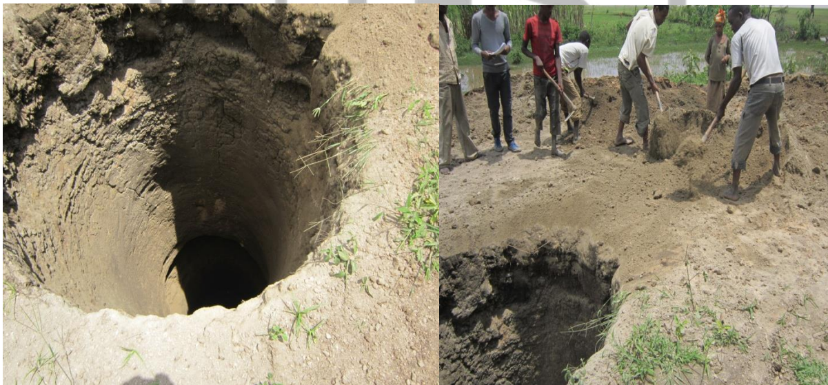
Figure 3.5 Borehole through goal Ethiopian and backfill
