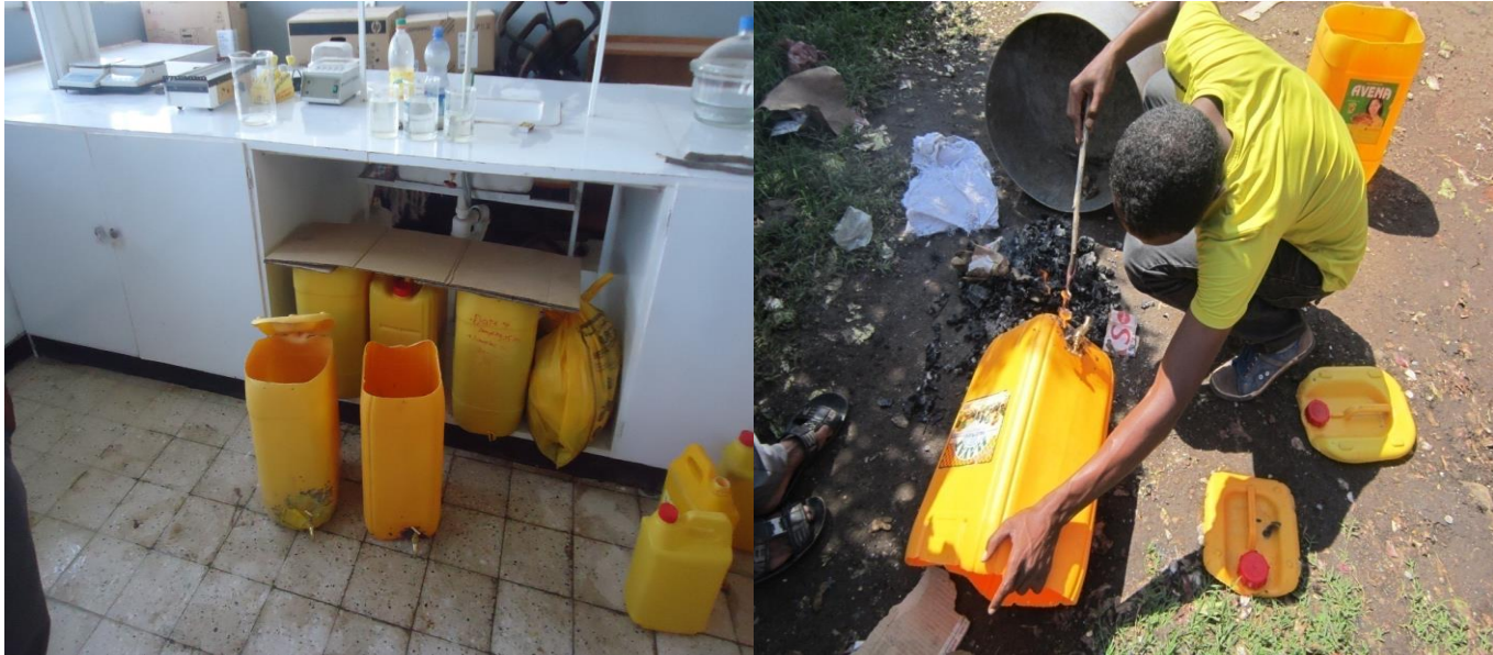
Figure 2.2 Bio-Sand Filter Containers (Jericans) Installation
