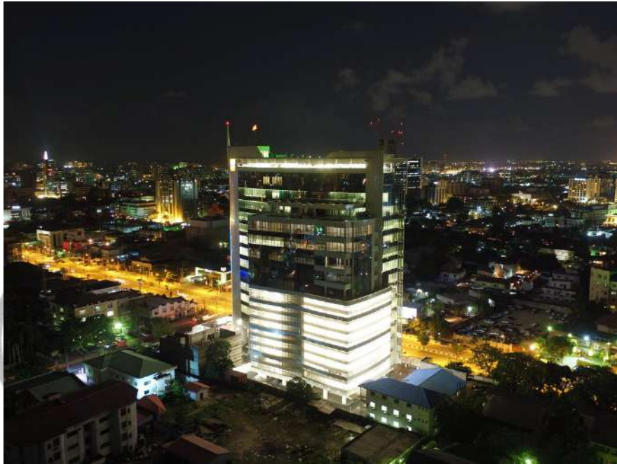
Plates 3.3: Rear view at night
