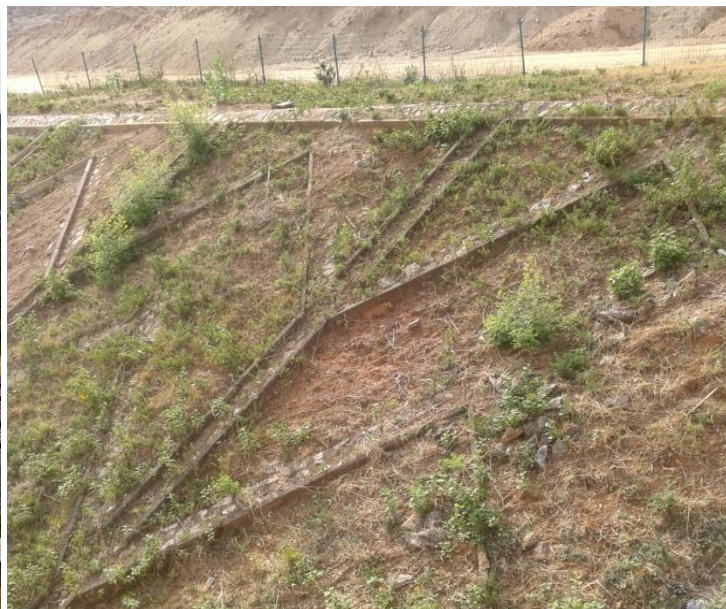
FIG.1b: Project Site with Herringbone System of Drainage
