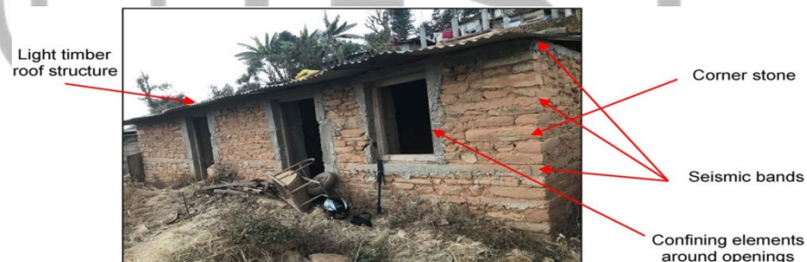
Fig 4.1: Stone masonry buildings in mud mortar
