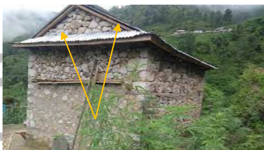
Fig 4.5: Stone masonry building with no gable wall
