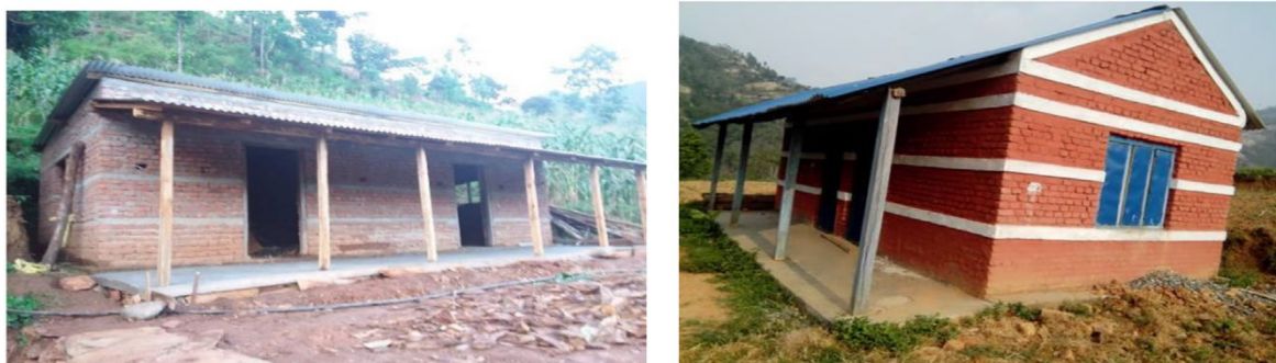
Fig 4.2: Brick masonry building in cement mortar.
