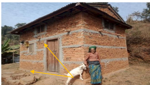
Fig 4.6: No sill band in attic level and improper band placement
