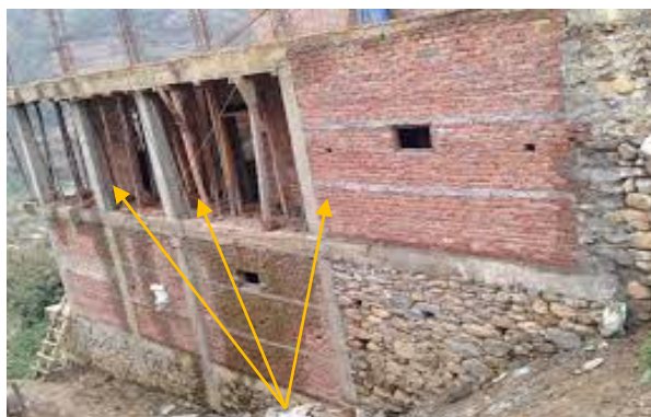
Fig 4.7: RCC building with 9x9 column
