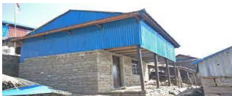
Fig 4.4: Hybrid structure with CGI covering at first floor
