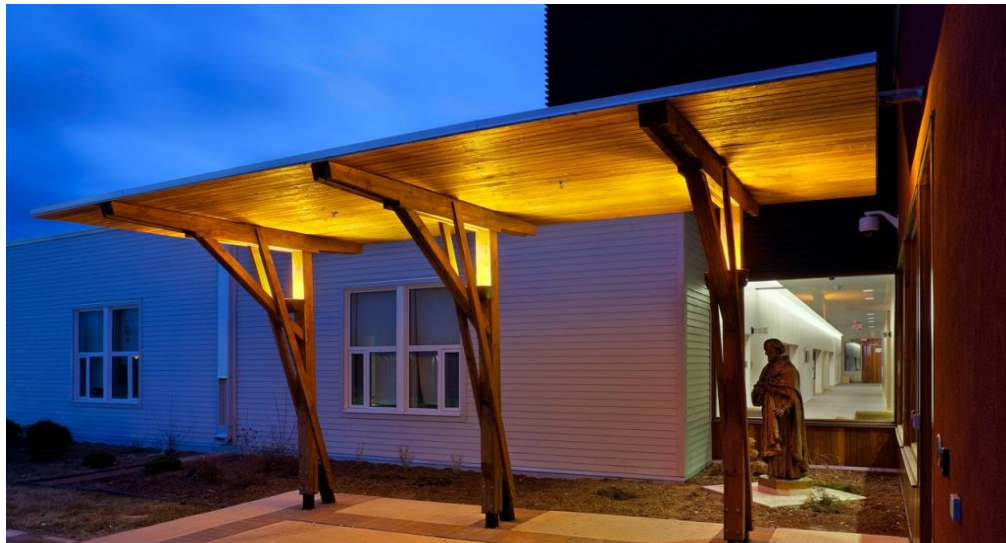
Fig. 4.5: The entrance to the facility
