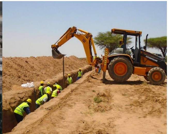
Figure 4.2 Water Supply Extension & Upgrading Project (Source: Field Survey 2019)
