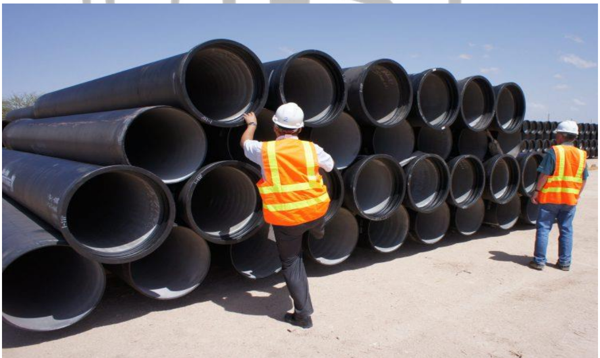
Hargeisa Water Supply Extension project pipe line Source: Field Observation
