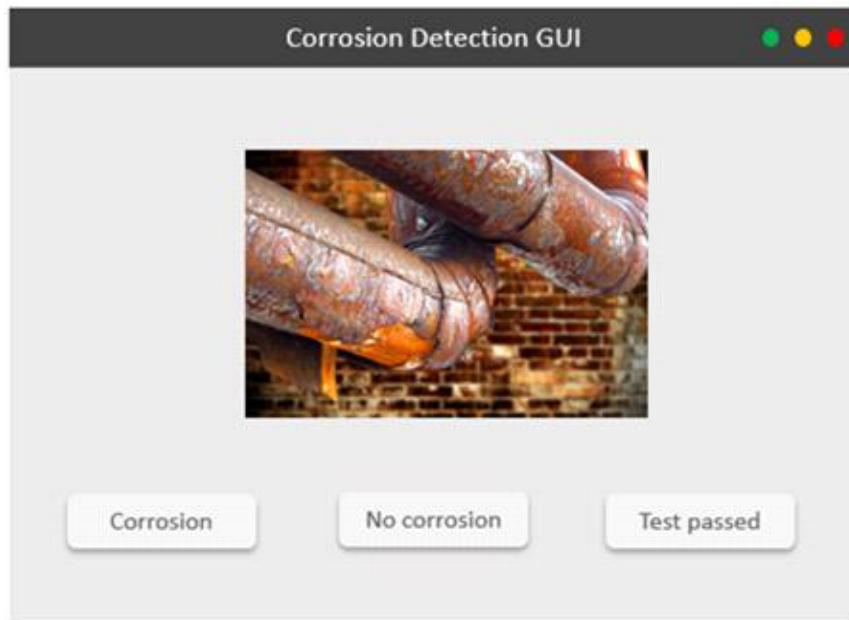
Fig 3: Corrosion detection GUI
