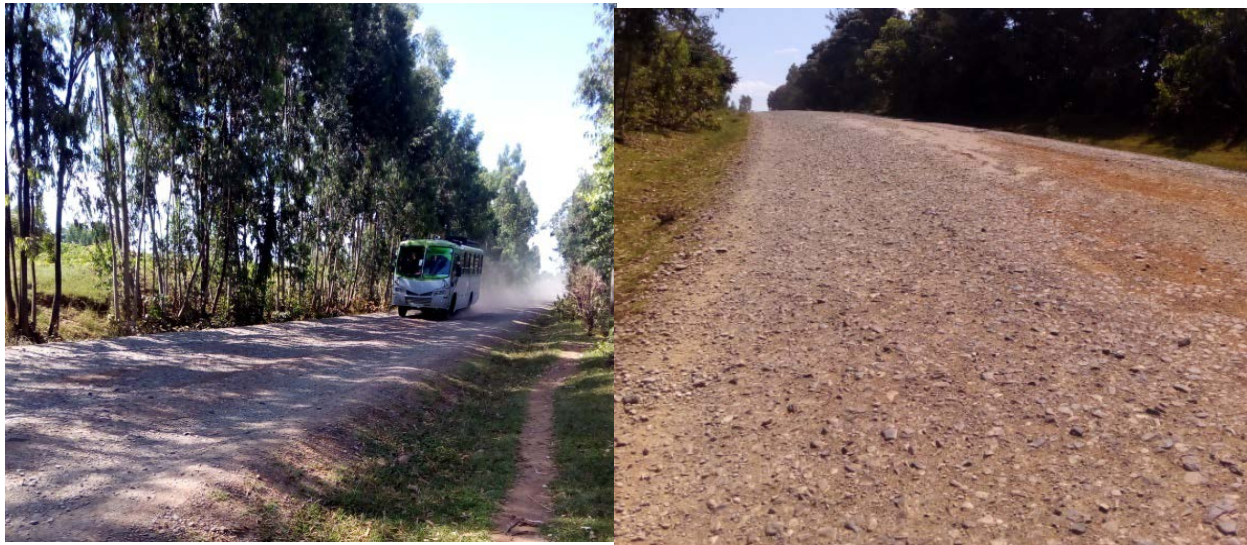
Figure 4 Dust in gravel road Figure 5. Stoniness in gravel road
