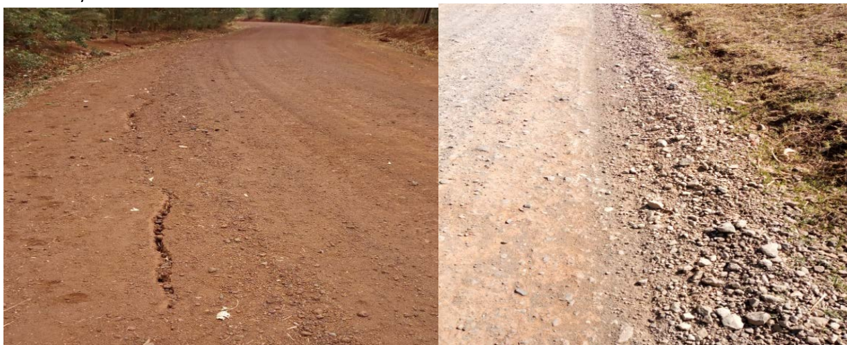
Figure 2 cracks on gravel road Figure 3 Ravelling on gravel road
