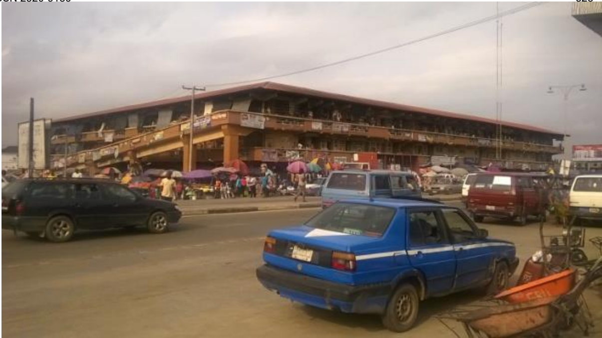
Figure 4. Exterior view showing ramp provided
