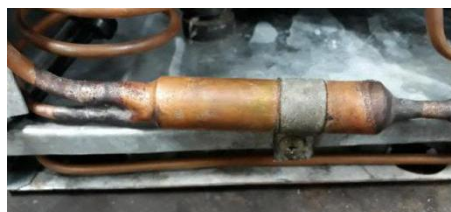
Figure 2.3 Copper filter drier
