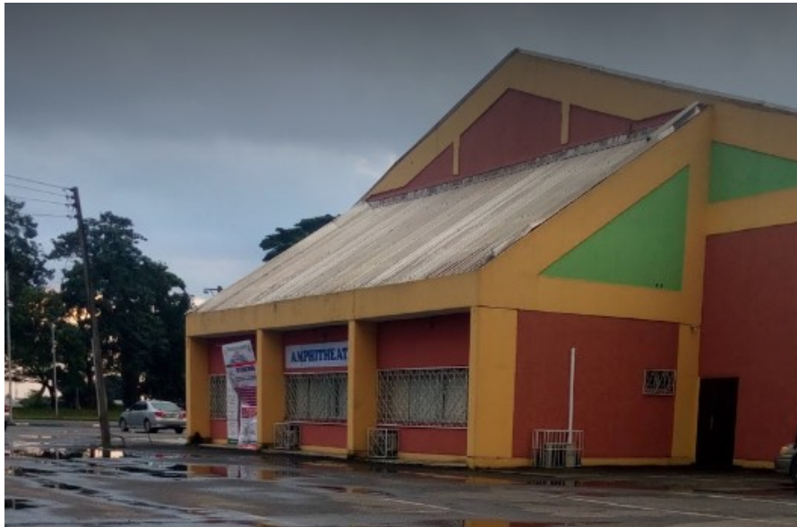
Fig 4.1: Amphitheatre Building with Poor Landscaping
