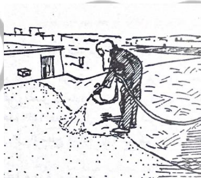
Figure. (4-D) : A layer of insulating material for concrete surfaces spread by a spray device
