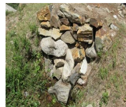
Figure 9: Undeveloped spring box of a sample water supply system
