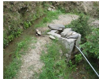
Figure 7: An inadequately engineered and unprotected source point
