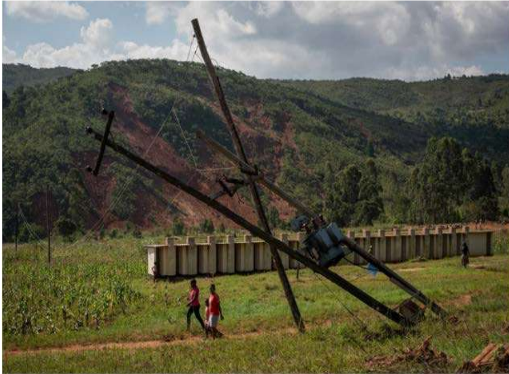
Figure 5: Destruction of Infrastructure for Crop and Food production.
