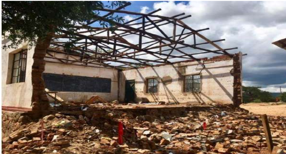
Figure 4: Early childhood development classroom block damaged by the Cyclone Idai, Chipinge District
