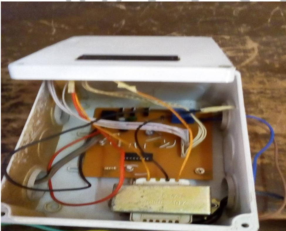
Picture of the exposed circuitry of the tap system
