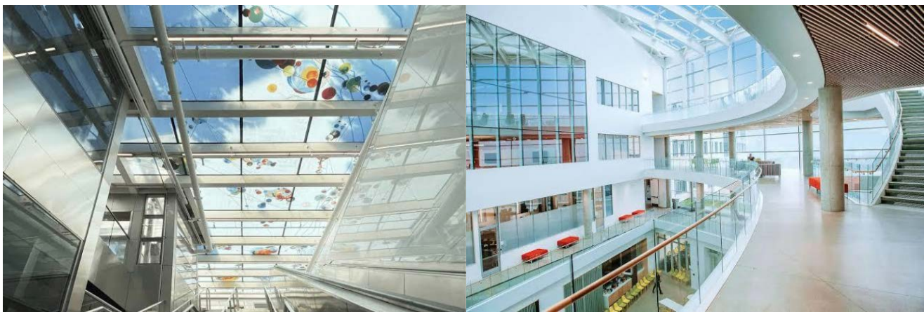
Figure 2.1: Skylight for Daylighting
