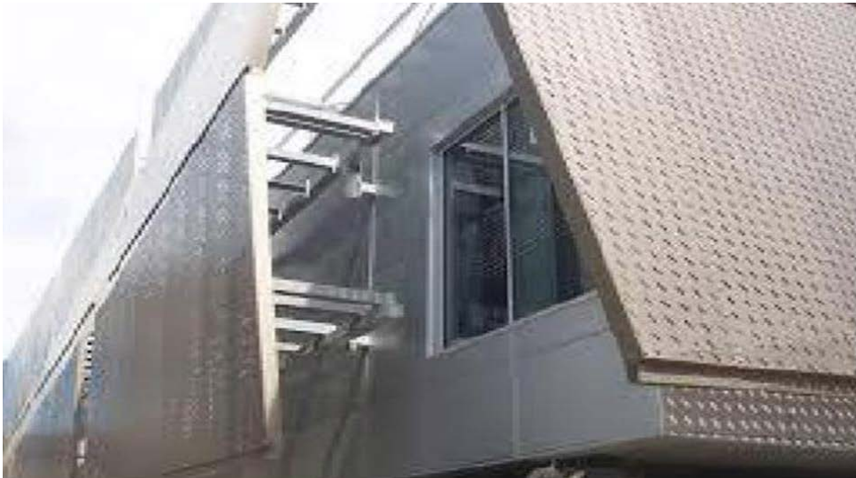
Figure 4.9: Showing Anodized Aluminum Cladding, a sustainability initiative
