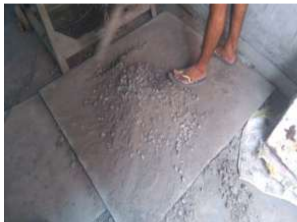
Figure 3: Mixing of coarse aggregate fine aggregate cement and silica
