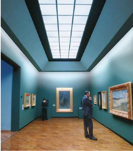
Fig. 5.0: Luminous ceilings are particularly suitable for painting galleries. The cove lighting provides additional brightness.
