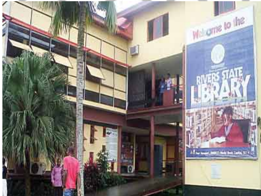
Fig. 7: Exterior view of public library Source: https://guardian.ng/saturday-magazine/rivers-public-library-deteriorates-questions-over-pharcourts-reign-as-world-book-capital/
