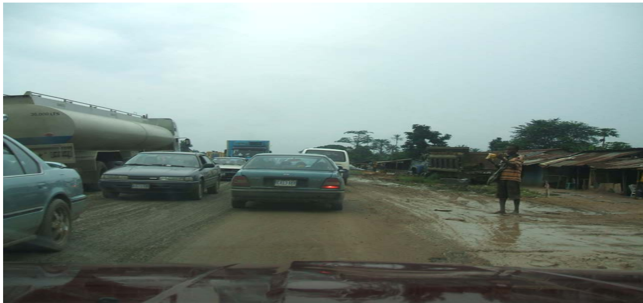
Plate 2: East-West Road Construction Induced Flooding and Traffic Site at Choba
