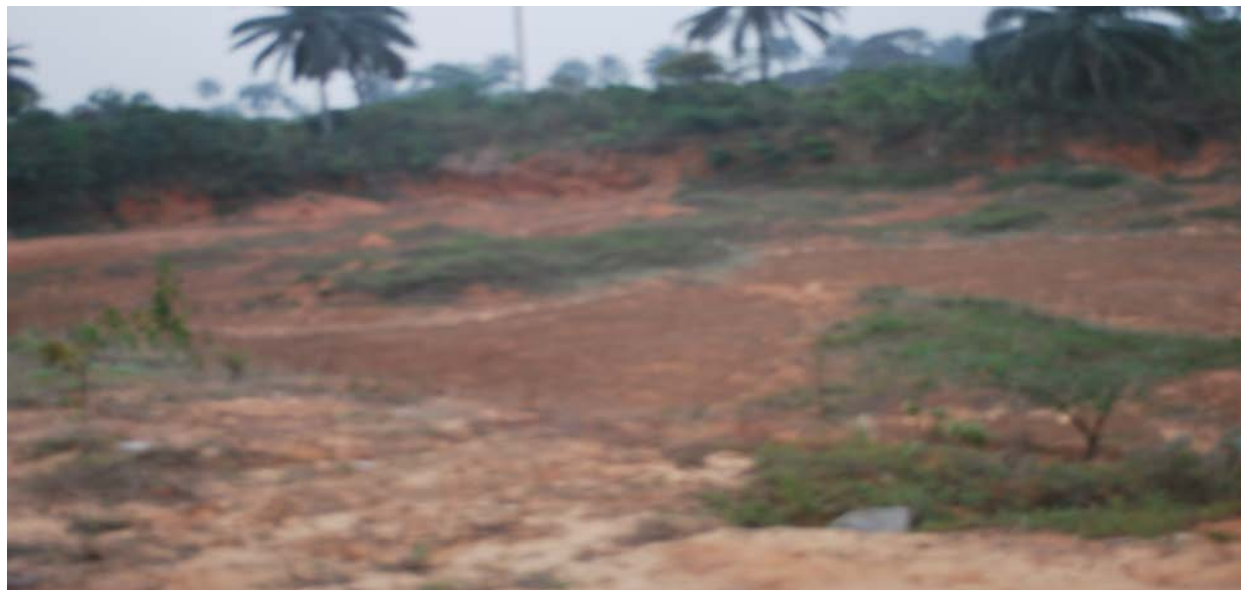
Plate 1: Road Construction Burrow-pit Induced Erosion Site along Elele Segment of the Road
