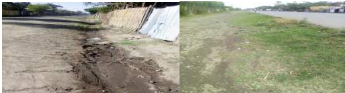
Figure 3.12: Effect of neglecting collector Drainage Systems around Lenda Ber(left side) and Mahal Arada (right side)
