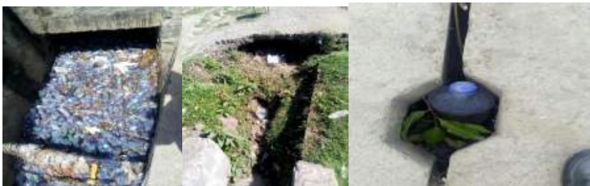
Figure 3.13: Blocked closed canal (right side), Blocked open canal (left side) and Damaged canal (middle)
