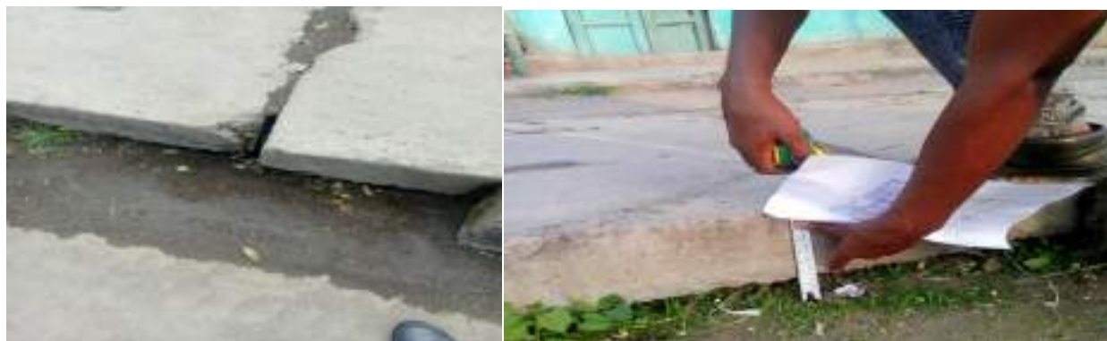
Figure 3.14: Manhole opening closed by garbage and less depth of opening
