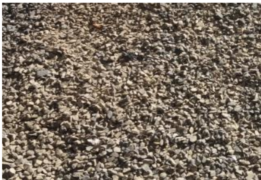
Figure 3.3. Coarse Aggregate with dust and clay particles
