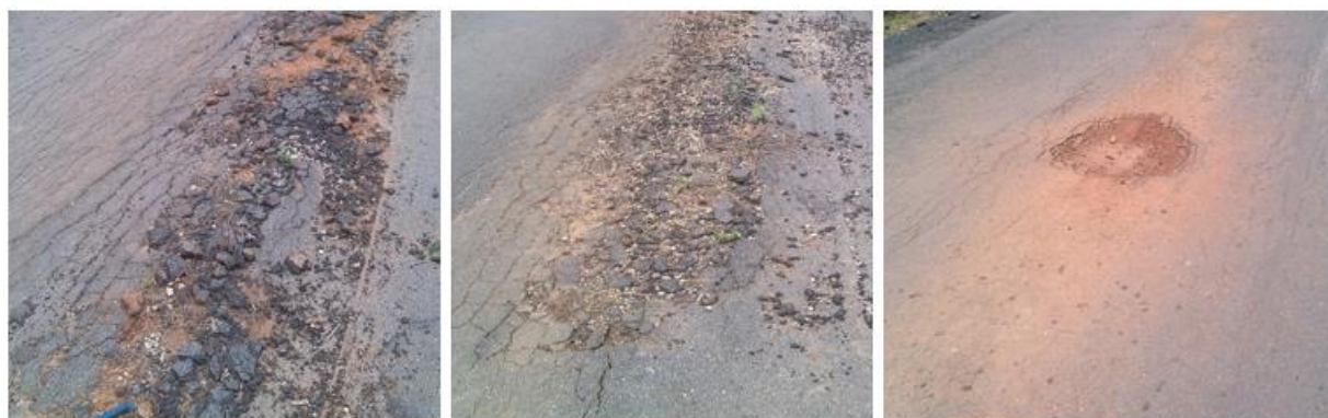
Plate 1.0: Shows the failed segment of the road.
