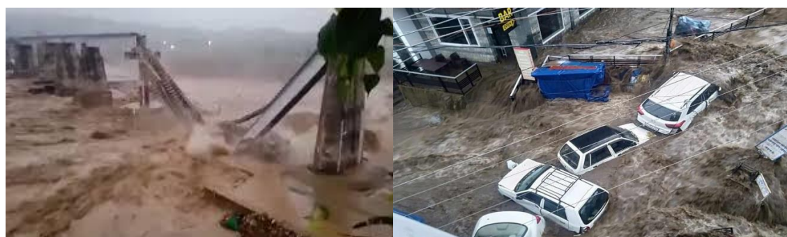
Figure 5 Collapse of Chakki bridge 2022, Figure 6. flash flood after cloud Burst in Dharamshala 2021
