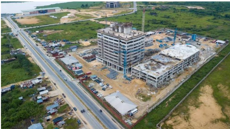
Fig. 6. CONSTRUCTION IN PROGRESS – AERIAL VIEW OF SITE
