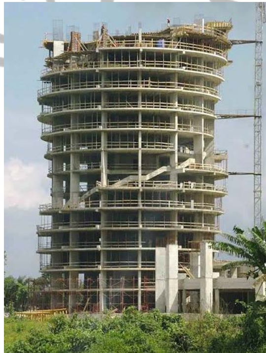
Fig. 10. THREE STAR HOTEL UNDER CONSTRUCTION – YENAGO
