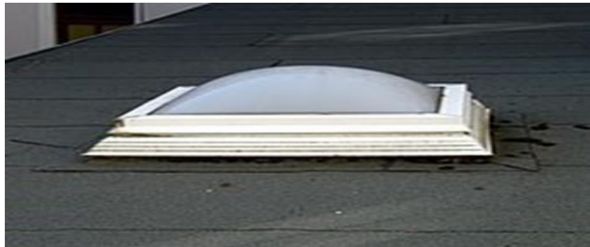
Figures 2.2.2: A Roof Lantern
