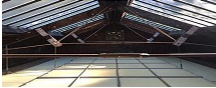
Figures 2.2.2.6: Skylights above laylights at the Lyme Art Association Gallery
