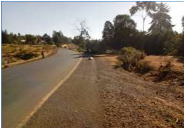
Figure 3.12 Chiri existing condition
