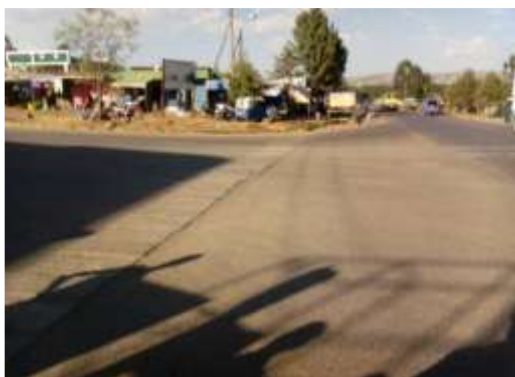
Figure 3.4 Gabriel Existing Road Condition
