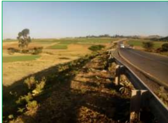
Fig 3.8 Wacan Mazoriya Existing Road Condition
