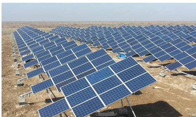
Figure 5 decentralized solar tracker.
