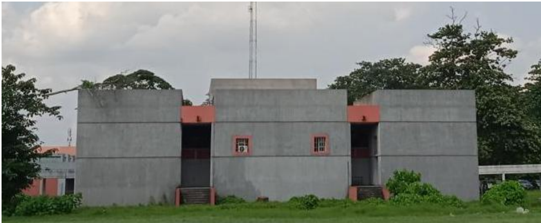
Plate 4.6: Rear view of the LT building, Rivers State University, Port Harcourt
