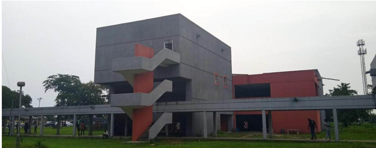
Plate 4.1: A perspective view of the LT building, Rivers State University, Port Harcourt
