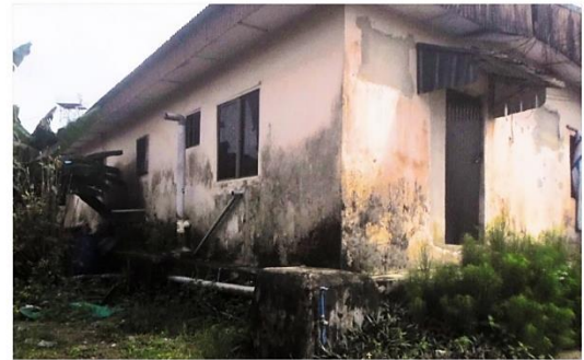
FLAKING, EFFLORESCENCE, FUNGUS GROWTH & RISING DAMP.
