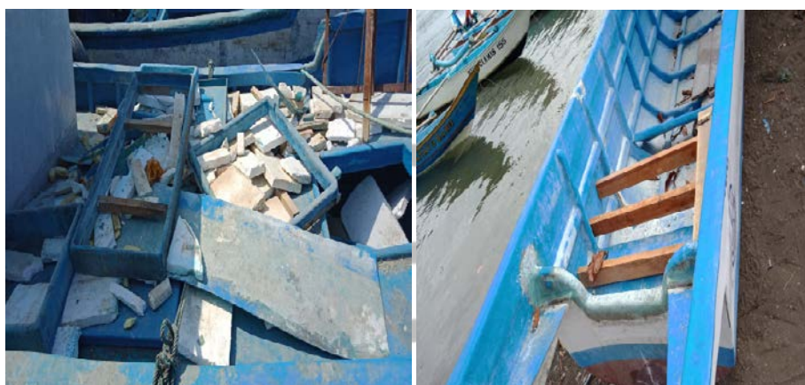
Figure 4 Grant vessel repair process
