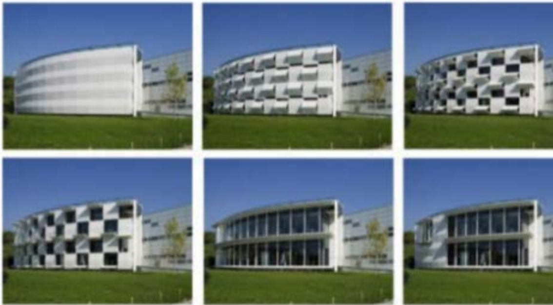
Figure 2.6: Example of Interactive Architecture, Kiefer technic showroom with façade itself is functioning as a shading device however given the users to manage the angle of the panel, and quantity of sunlight transmitted into the interior space.
