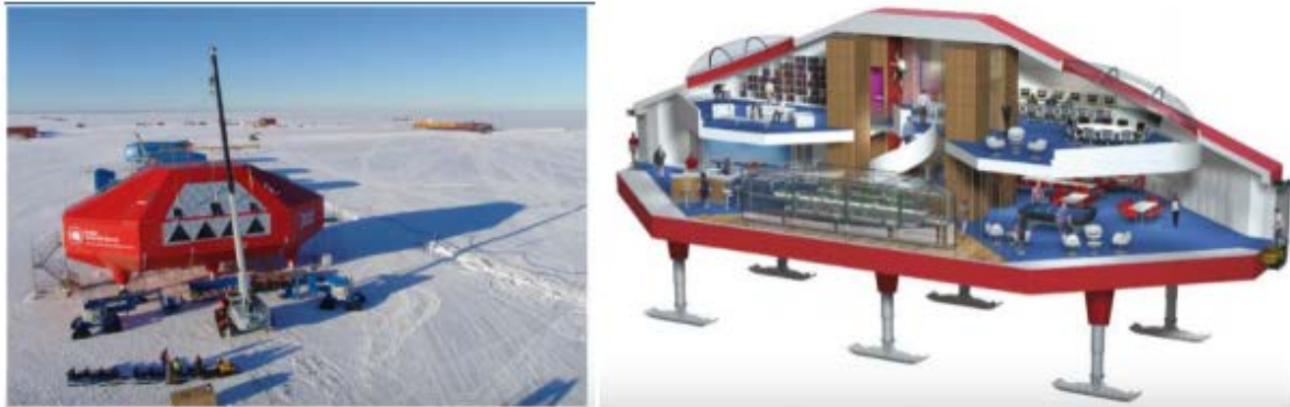
Figure 2.4: Example of Mobile Architecture, Halley Vi Antarctic Research Station, that became Mobile Home for 50 Scientists at Antarctic
