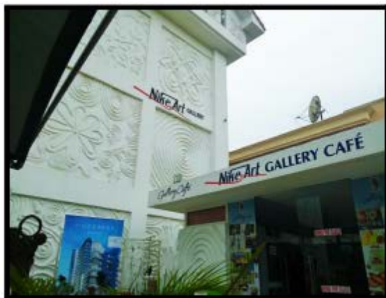
Figure 4.7: Approach View of Nike Art Gallery Centre
