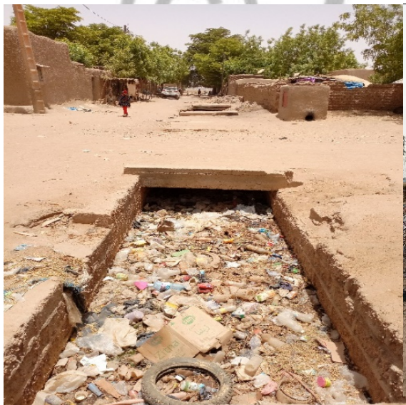
Photo 3: Main drainage ditch filled with garbage
