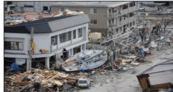
Fig 1.1: Collapsing the brick masonry structures in Tohoku, Japan due to Earthquake 2011 ( http://nehrpsearch.com )
