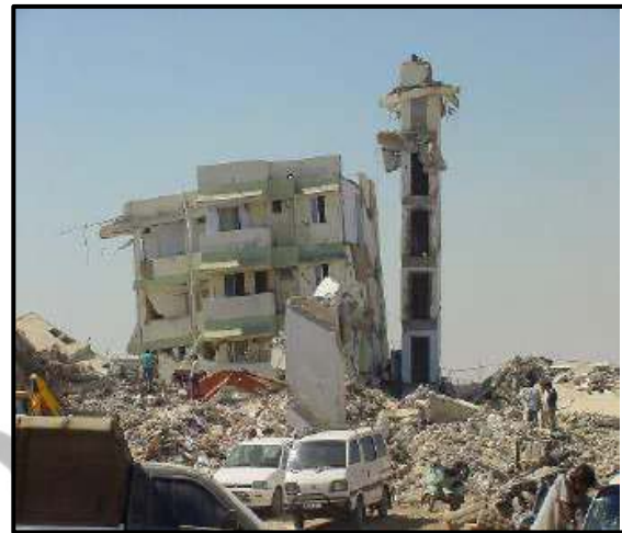
Fig 2.2: Apartment collapse in 2001 Bhuj earthquake with separation of the lift shaft ( www.bbcnews.com/exclusive_photage )
