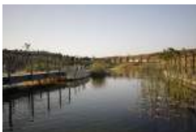
A retention basin for periodic floods will be excavated, where ramps and bridges connect to the plain
