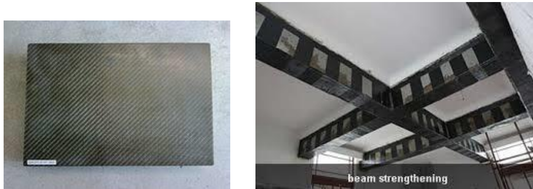
Figure 3.34: (a) CFRP strip, (b) Application of CFRP [2].
