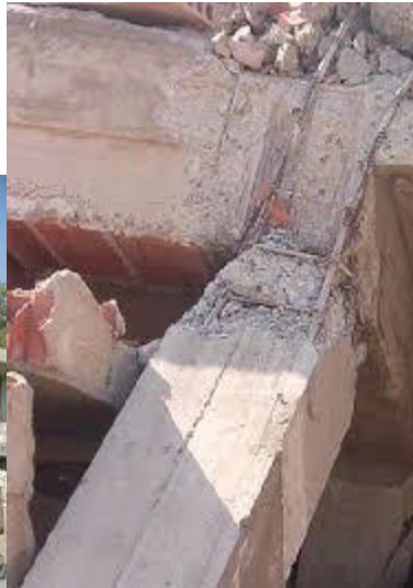
b)beam column joint failure
