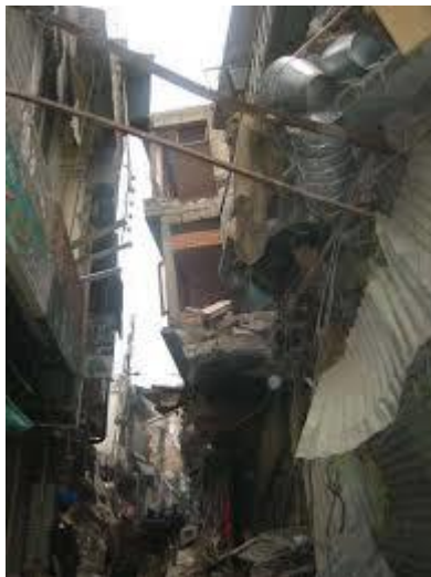
a)soft story failure
