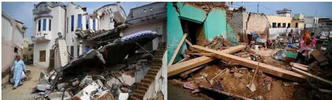
a) Reinforced concrete construction(pucca) b) stone masonry construction(katcha)
