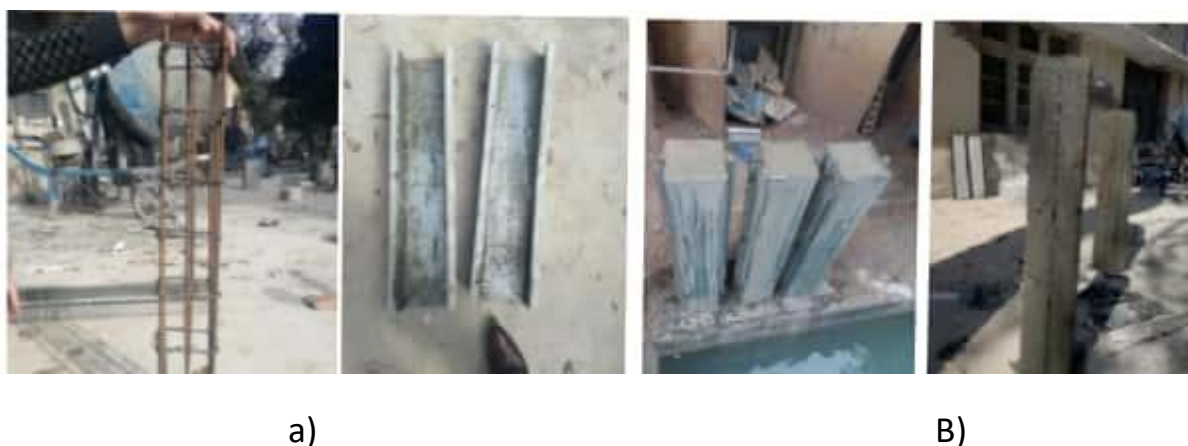
Figure 3.9: (a) Transverse and longitudinal steel, (b) Casting of RC column
