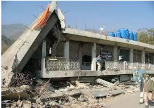
a)soft story failure
