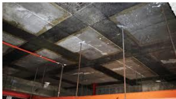
(b) Application of CFRP in Residential Apartments
