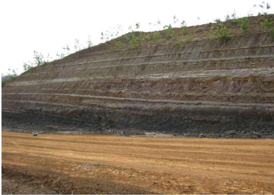
Fig. 2: Outcrop of Ahoko-Ebira (location 1) showing the dipping direction
