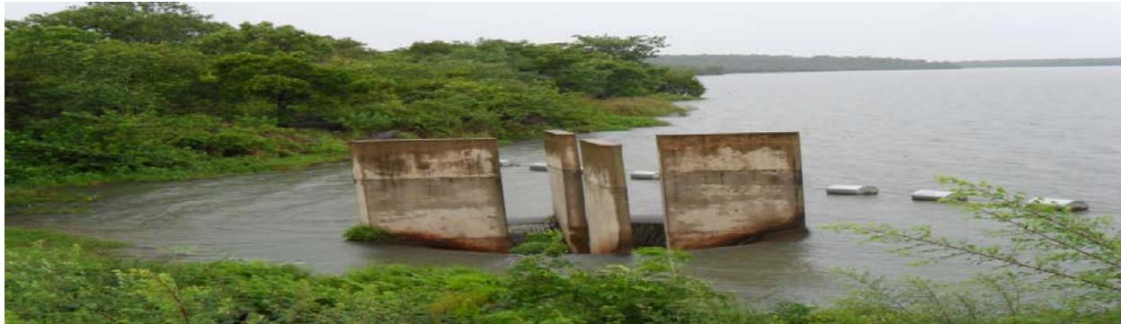
Plate I: Doma Dam Showing Morning Glory and Open Channel Spillway
