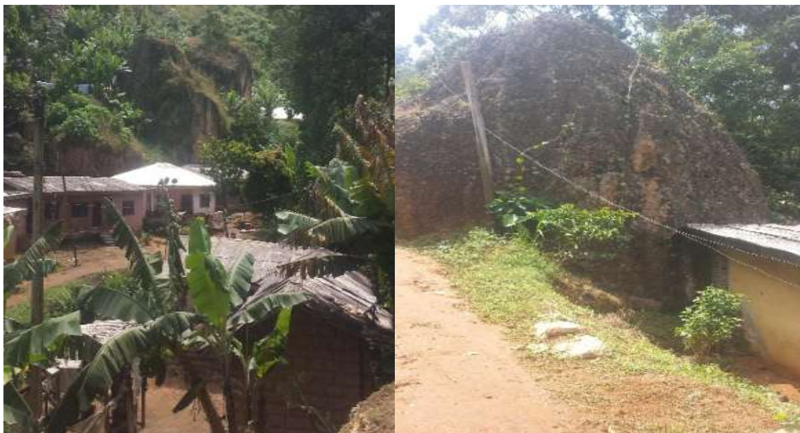
Fig 6a: Construction of houses around rock fall zone at Sisia III-Nkwen
