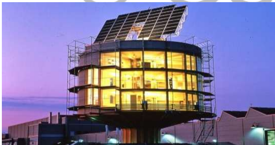
fig 5.1.1: The spinning, sun-chasing Heliotrope designed by Rolf Disch. It can generate up to five times as much power as it needs to operate. The home sports a giant angled solar array on the roof and the entire structure is mounted on a pole timed to rotate 180 degrees each day as it follows the sun.
