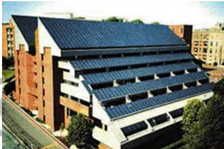
Figure 9. Building Integrated Photovoltaic Panels [BIPV]
