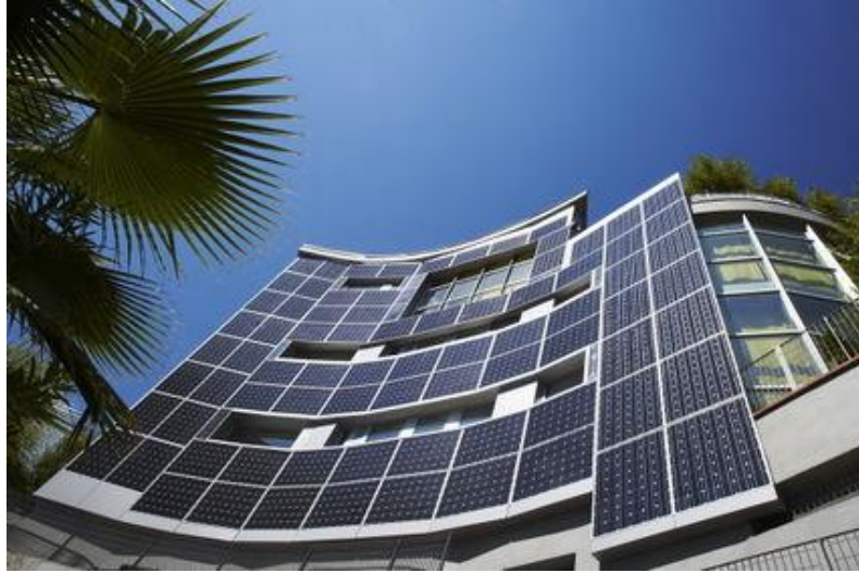
Figure10 Building Integrated Photovoltaic Panels [BIPV]
