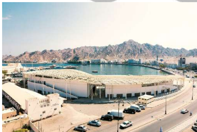
Figure 3. On Site photos of Muttrah fish market. Source. https://snohetta.com
