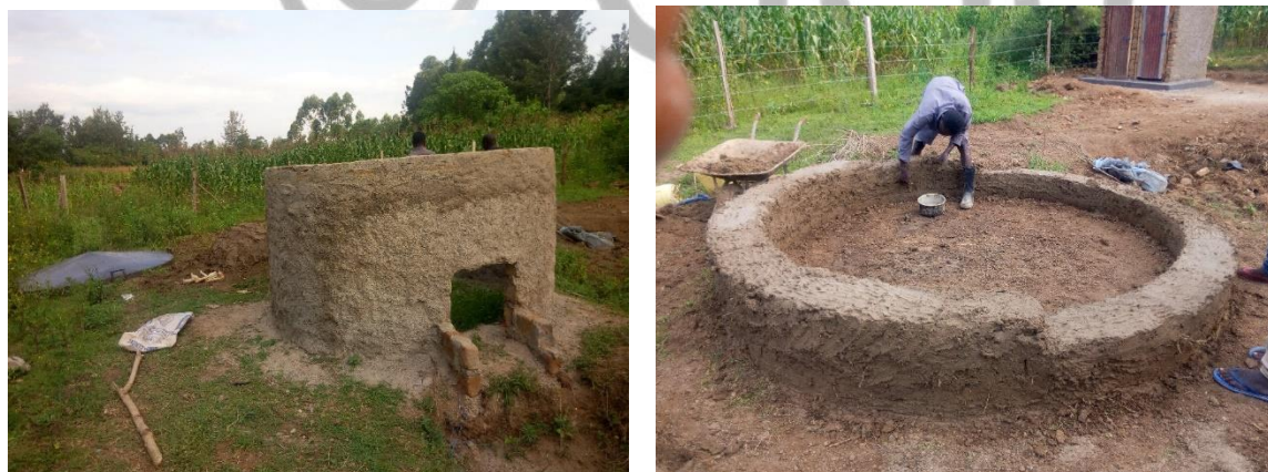
Pyrolysis chambers made of Bricks and clay walls with a metallic cover
