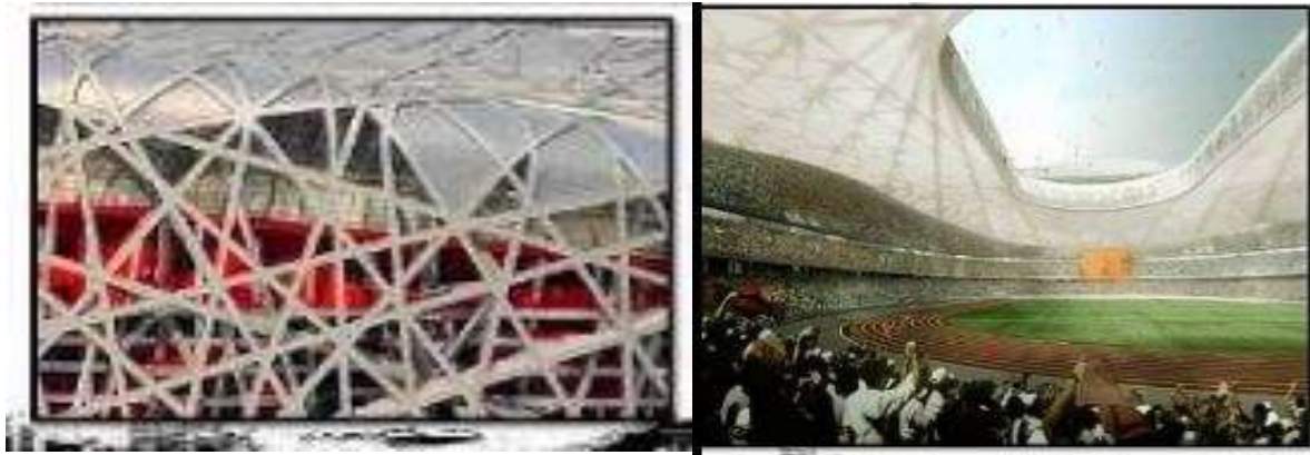
Fig. 5 Sustainability in the building. Photo: Ali Bacharouche Sadek Saad
