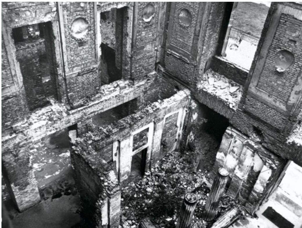
Figure 12: Destruction after fire
