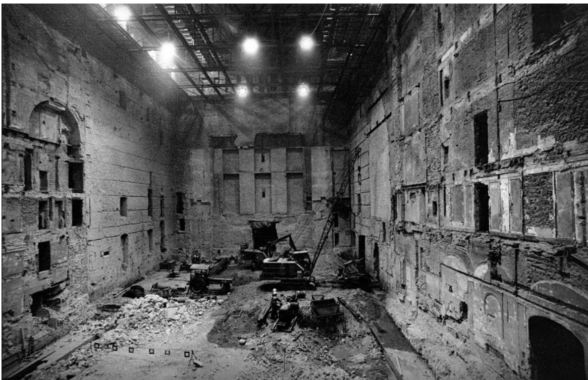
Figure 14: Demolition and clearing works for the interior
