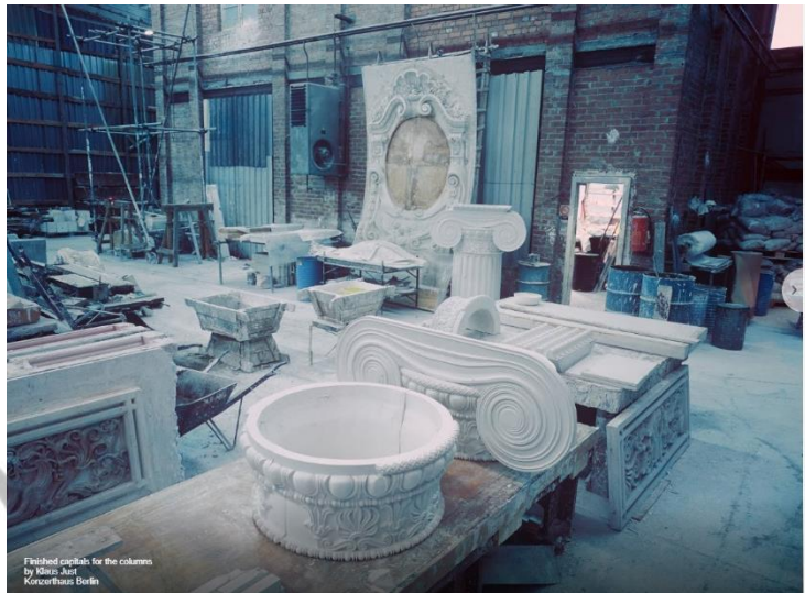
Figure 18: Stucco formwork at site
