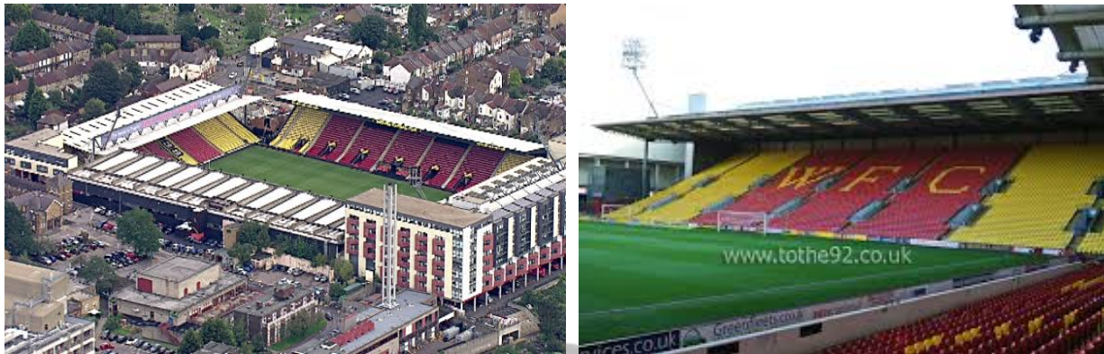
Fig3. Watford Stadium with translucent PVC. Vaulted shell roof cover. Source; internet
