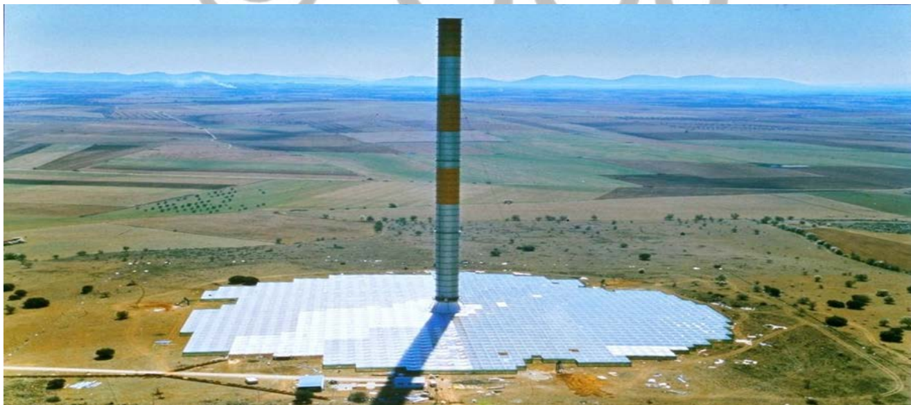
Figure 6 "Manzanares solar chimney power plant"
