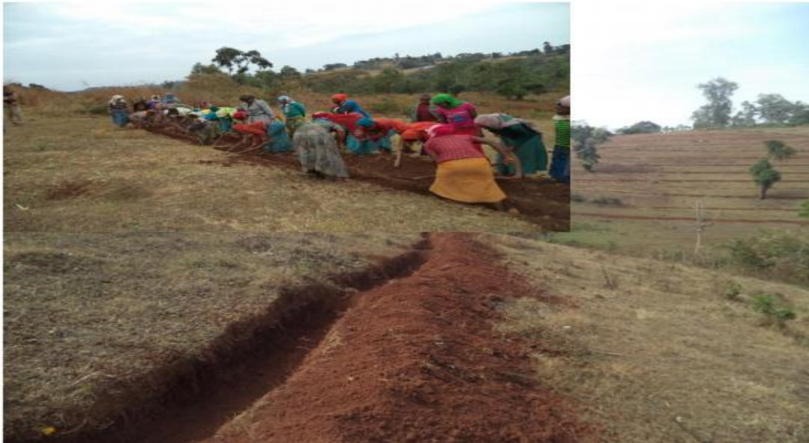
Fig. 4.12 Field photograph, Soil bunds, 2018
